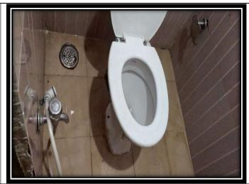
Poor waterproofing in the toilet. The toilet seat pipe is not cemented properly, a big gap is visible.
