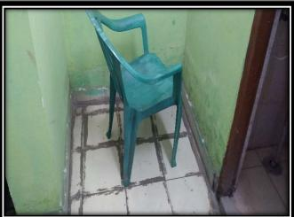
The floor near the toilet is not cemented well therefore whenever the water flows out of the bathroom or during cleaning, water percolates through the gaps.
