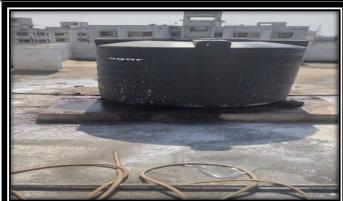
Although the storage tanks are kept on a high surface the adjacent areas are not made to drain away the overflowed water
