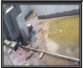
Due to continues water logging at the site of the water storage tank, the mould has developed making the surface uneven to flow the water
