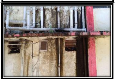
The newly instated pipe also has a similar problem of leaking at the joints, the plumbing is very poor.
