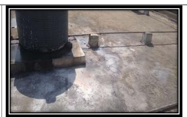
The overflow of a storage tank at the terrace always keeps the terrace floor wet.
