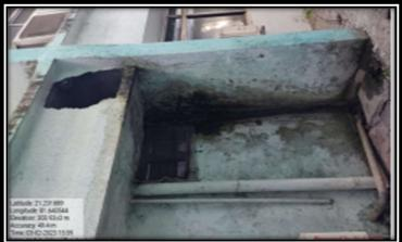
Toilet area drainage pipes leakage at the joints
