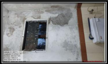
Water supply pipe leakage in the wall
