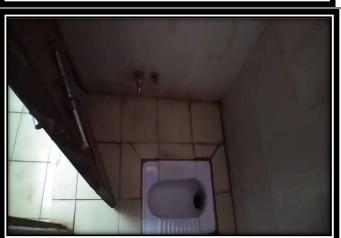
The water tab in the toilet, washing area, and bathroom is leaking all the time making the cracked floor ideal for seepage
