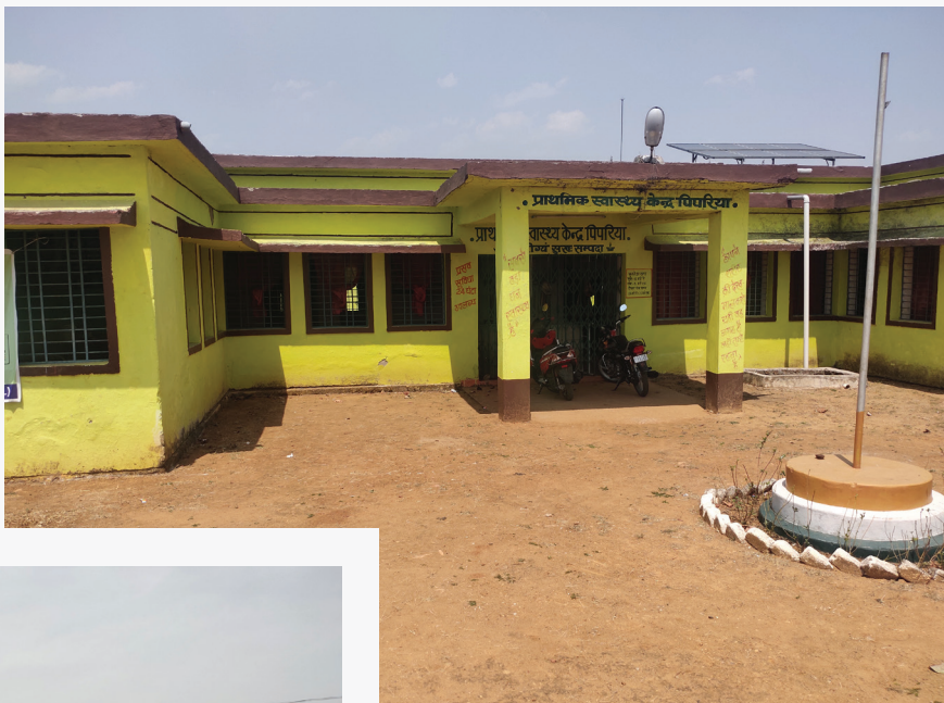
The health facility is highly prone to heat with no trees and green areas around it.
